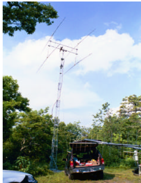
To the left is the two meter SSB array atop a crank up tower. Four beams are harnessed together into a phased array. The booms of each antenna are 31 feet long.
