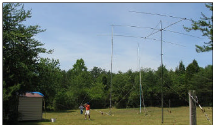
Setting up in the final hours required putting up the four-square array and a beam on a surplus military tower. Oh, and don't forget the sunshade for the SSB hut.
