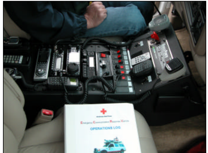
Even the driver has a well-equipped workstation. Numerous hand-helds are packed in equipment boxes stowed in the cargo space.
