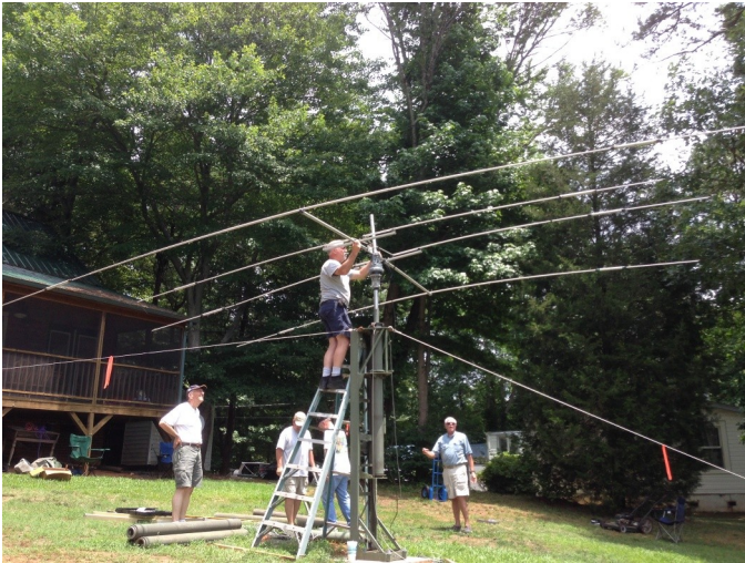
Here's Alex, KJ4IEC, putting the TA33 on Chris' crank-up military surplus mast, under close supervision. A special thanks to Alex, who, even though he isn't a CDXA member, gave us a lot of help during setup, and operation.
