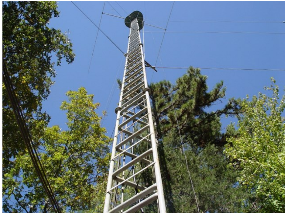
Antenna just to the right near top
